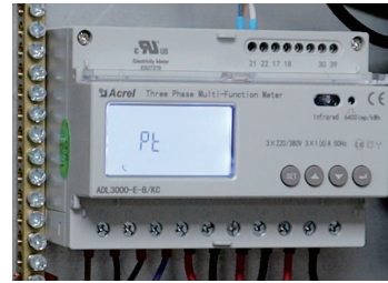
Figure 4.25 PT or CT Ratio Setting
